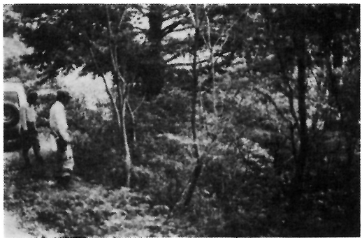
Photo. 12 Experimental plot No.6 on banking slope of forest road construction in 1975 (Oct. 6, 1985)
