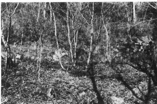
Photo. 11 Experimental plot No.6 on banking slope of forest road construction in 1975 (Dec. 5, 1984)
